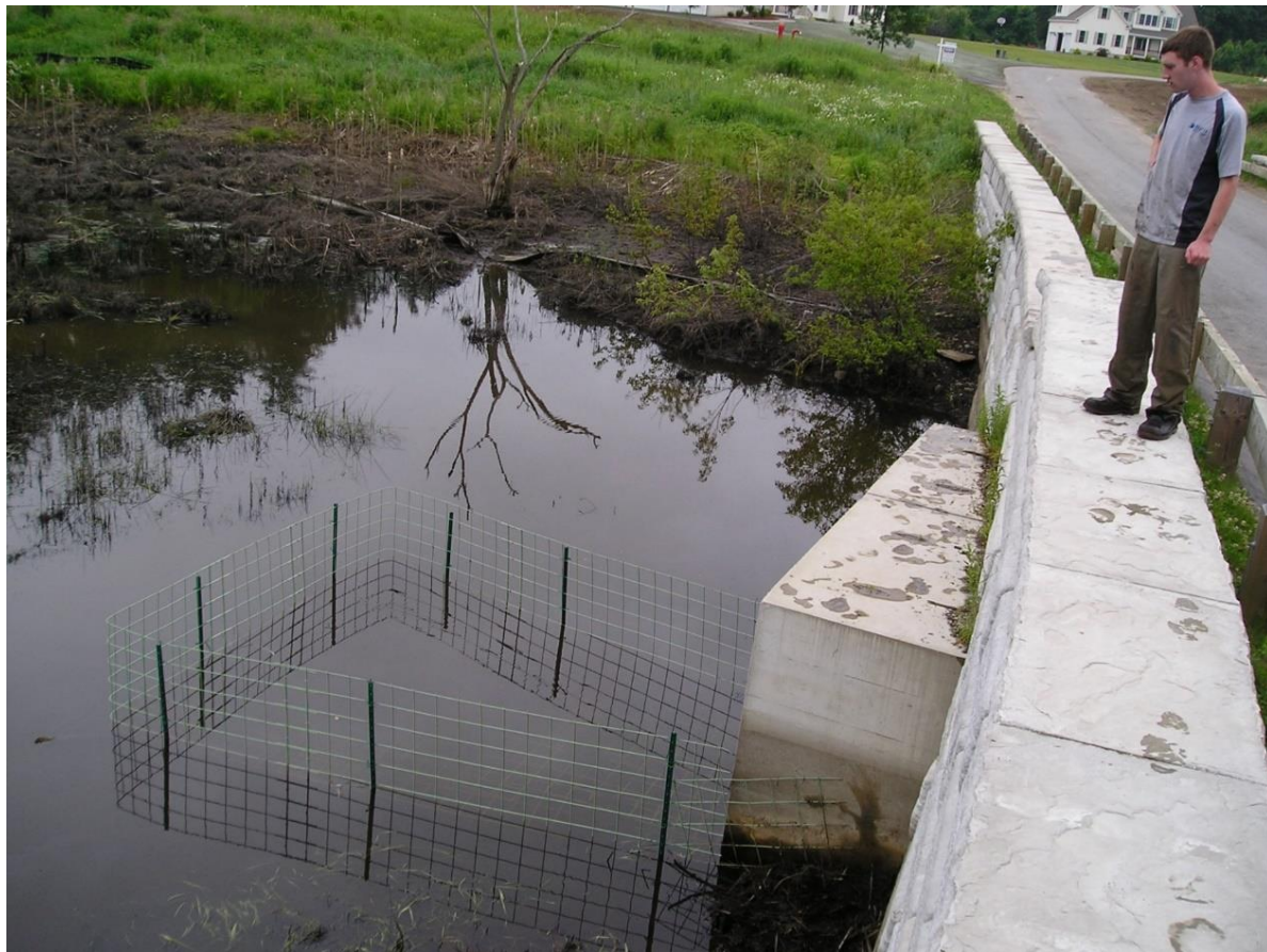
Figure 16. Trapezoidal fence to protect culvert in Massachusetts. Photo by Michael Callahan ( www.beaversolutions.com ).
