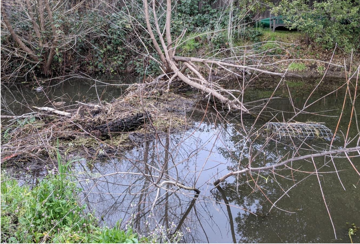
Figure 14. Pond leveler device - caging around intake visible above a dam.
