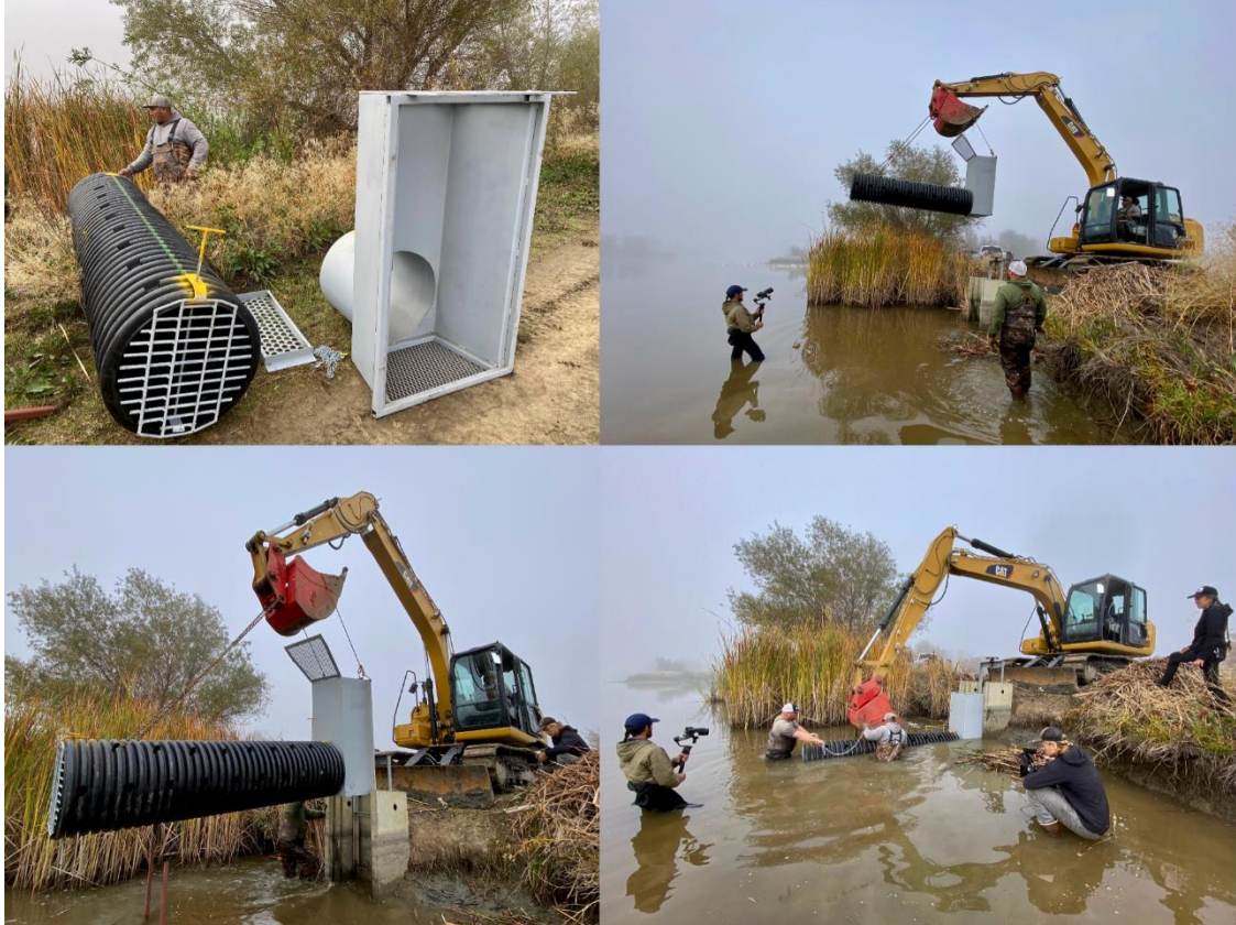
Figure 17b. Weir inlet protector device installation. Courtesy of OAEC.
