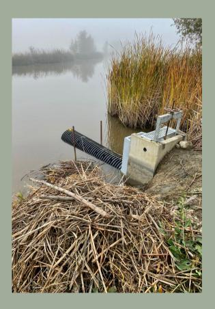
The Beaver Back Saver eliminates the constant clearing out of twin track weirs from beaver activity. The retrofit slides on to an existing weir, drawing water through a perforated pipe, capped with a metal grate, allowing it to convey water without beavers hearing or sensing the flow, thus deterred from plugging it up.
