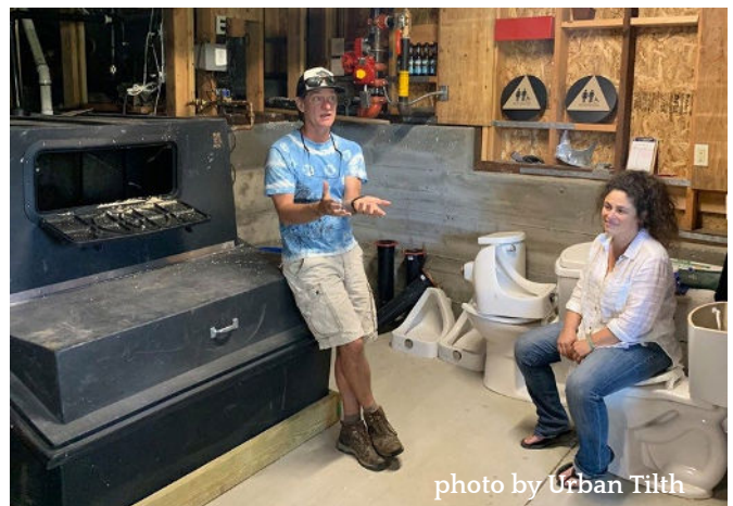
OAEC staff showing the Clivus Multrum composting unit to the Urban Tilth community underneath the new meeting hall.
