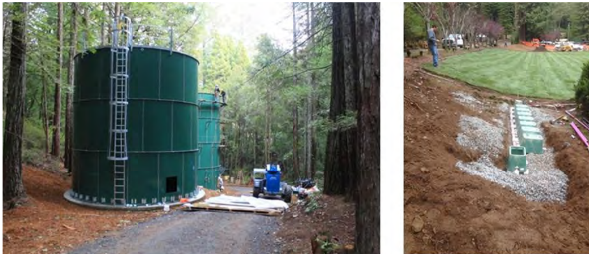
Figure 51. Westminster Woods Project. Left: Two tanks (total capacity 175,000 gallons) which store winter water to irrigate the camp's playing fields in the summer; Right: Valves installed as part of the new irrigation system.
