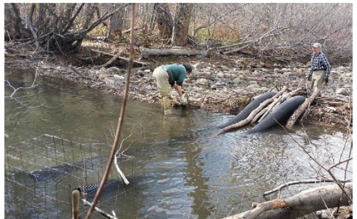
Sherry and Ted Guzzi of the Sierra Wildlife Coalition install a flow control device on Taylor Creek in South Lake Tahoe. NOTE: We are sad to report that since the writing of this guidebook, Ted Guzzi has passed away. His passion and dedication to beavers will be dearly missed. (Photo: Sheri Harstein)
