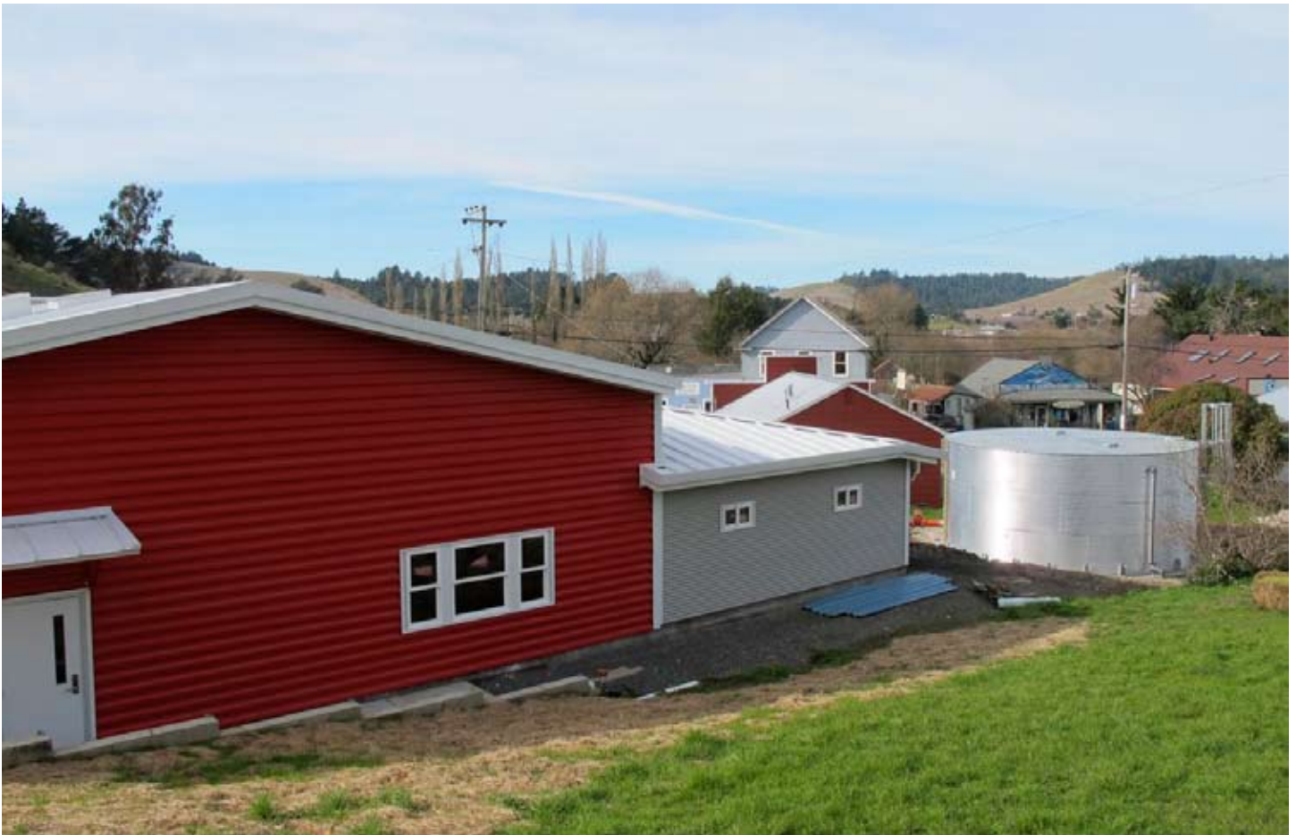
Rear view of the new Bodega Volunteer Fire Department and its roofwater harvesting storage tank installed by the SOS program in Bodega, CA
