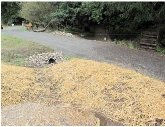
Overflow goes through culvert to second sediment basin on other side of the road
