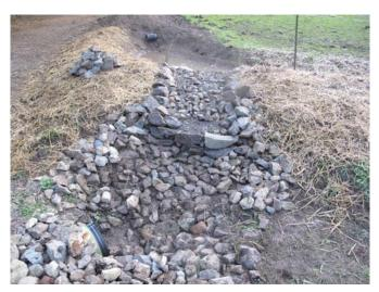
Rockwork for overflow prevents erosion
