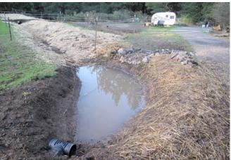
Finished sediment basin and swale with overflow
