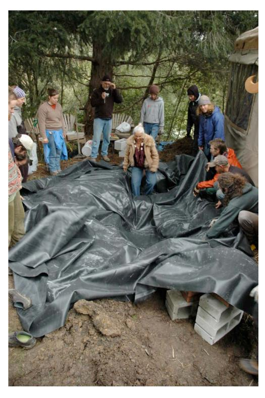
on top of them. Having the liner under this feature will ensure that any spillover or leakage from the flow forms will drain back into the pond. The spaces between the cinder blocks will be back filled with lava rock and plants in potting tubes will be planted into this medium to take advantage of this extra source of moisture and provide additional bio-filtration.
