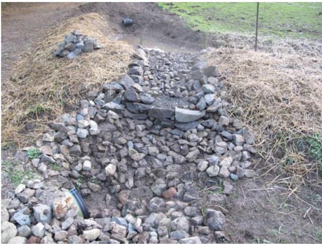
*Rockwork for overflow prevents erosion*
