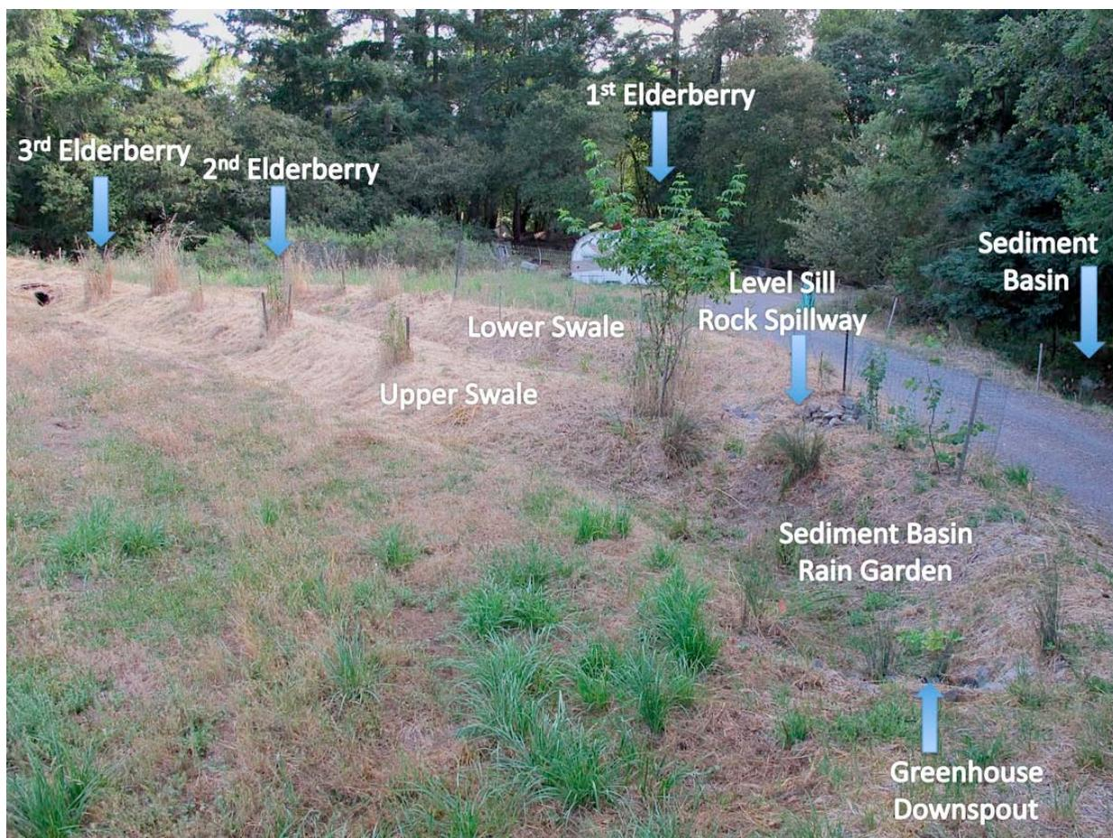
Figure 2. Image of the sediment basins and swales planted with California natives as of July 2012
