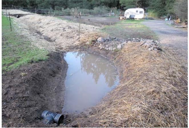
*Finished sediment basin and swale with overflow*
