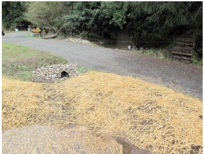
*Overflow goes through culvert to second sediment basin on other side of the road*
