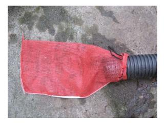
To prevent any debris from getting into the tank we wired this reused plastic onion sack onto the end of the pipe. After three winters of operation, we found no more than 25 leaves in this filter. This is a low cost solution that reuses an existing resource (onion sack) that might otherwise be tossed into the landfill.
