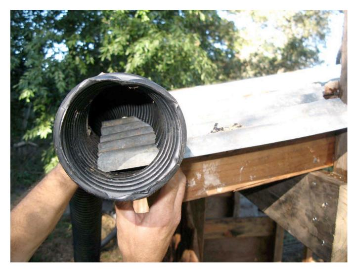
Here you can see the cross section of the pipe over the edge of the roofing. We made sure to let the roofing overhang about 3-5" to allow space for the drainpipe to slide over the edge. Here you can see how we left the first four inches uncut to allow for an end cap.
